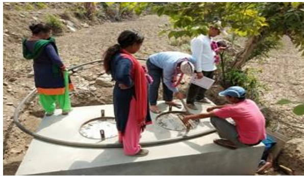
Figure 3 PSO & RM level WUG chhachara Monotring At Lanakedarshwar
